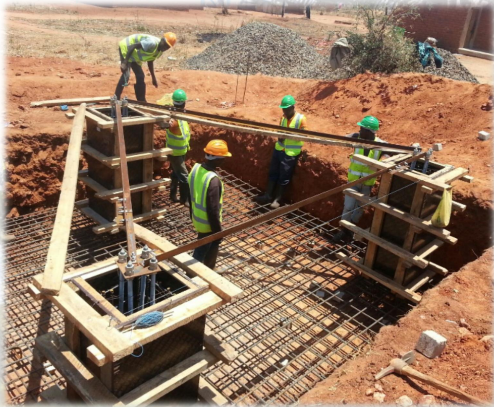
Formwork Installation
