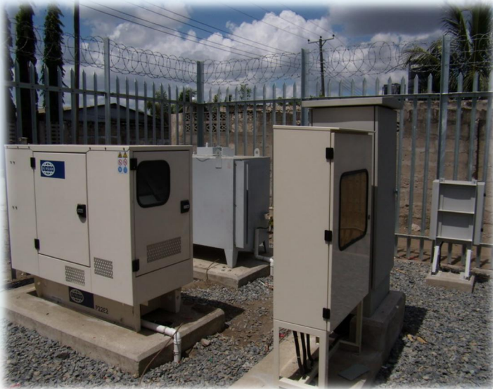
Installations of Tower generators and power room (shelters)
